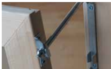
Windows with double closing system and tilt and turn opening system, except for horizontal fixed windows
