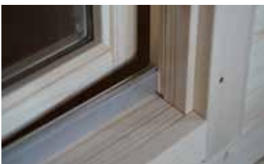
UK DGP+ windows are supplied with an Aluminium water gutter as standard to prevent water from entering
