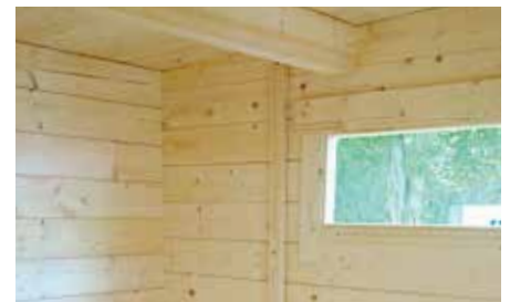
Wooden storm strips or threaded rods (depending on model) protect your garden cabin against strong winds
